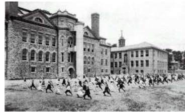
Ardmore Avenue School built in 1875, destroyed by fire and re-built in 1900, served Ardmore students until 1963.
